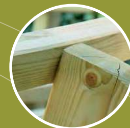
Wood cracks
